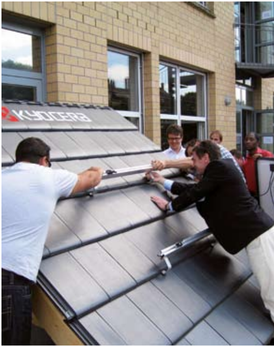
Men at work – Modulmontage am Demodach
